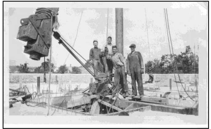
Construction workers in 1922 Photo contributed by Harold Regan.
